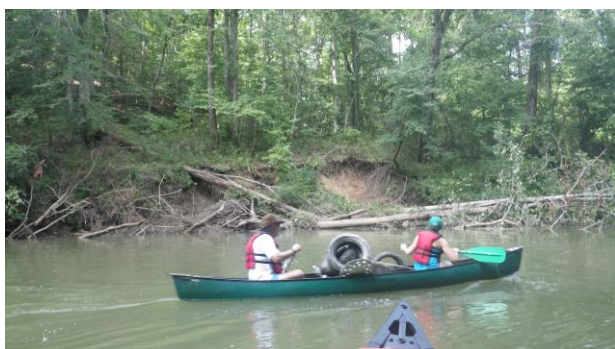
July 29, 2017. A new bank collapse adjacent to an old collapse. Note that leaves are still on the tree, indicating this is a recent event.
